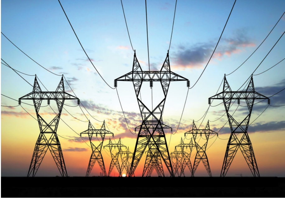
Figure 5: AC Transmission Lines
